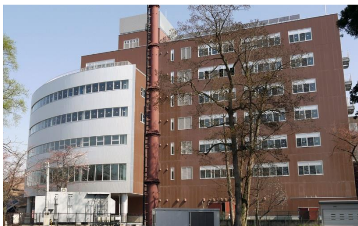
Outward Appearance of Frontier Center for Organic Materials
